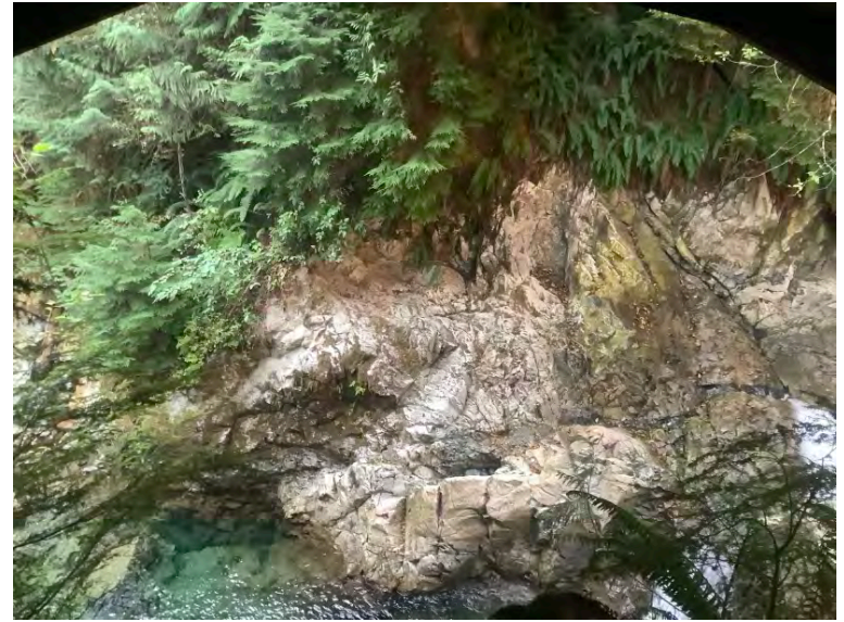
Right Bank Abutment when facing downstream
