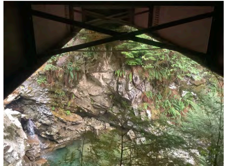
Left Bank Abutment when facing downstream
